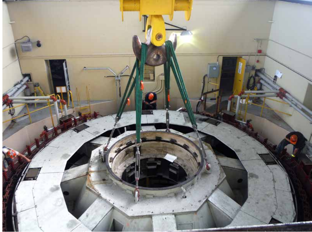
Hoisting an upper bracket at the Niagara Pump GS.
