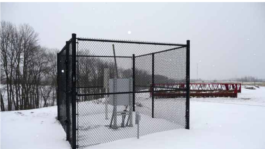
Air monitoring station for the Darlington environmental monitoring program
