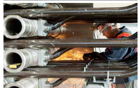
Welding at the Darlington Energy Complex
